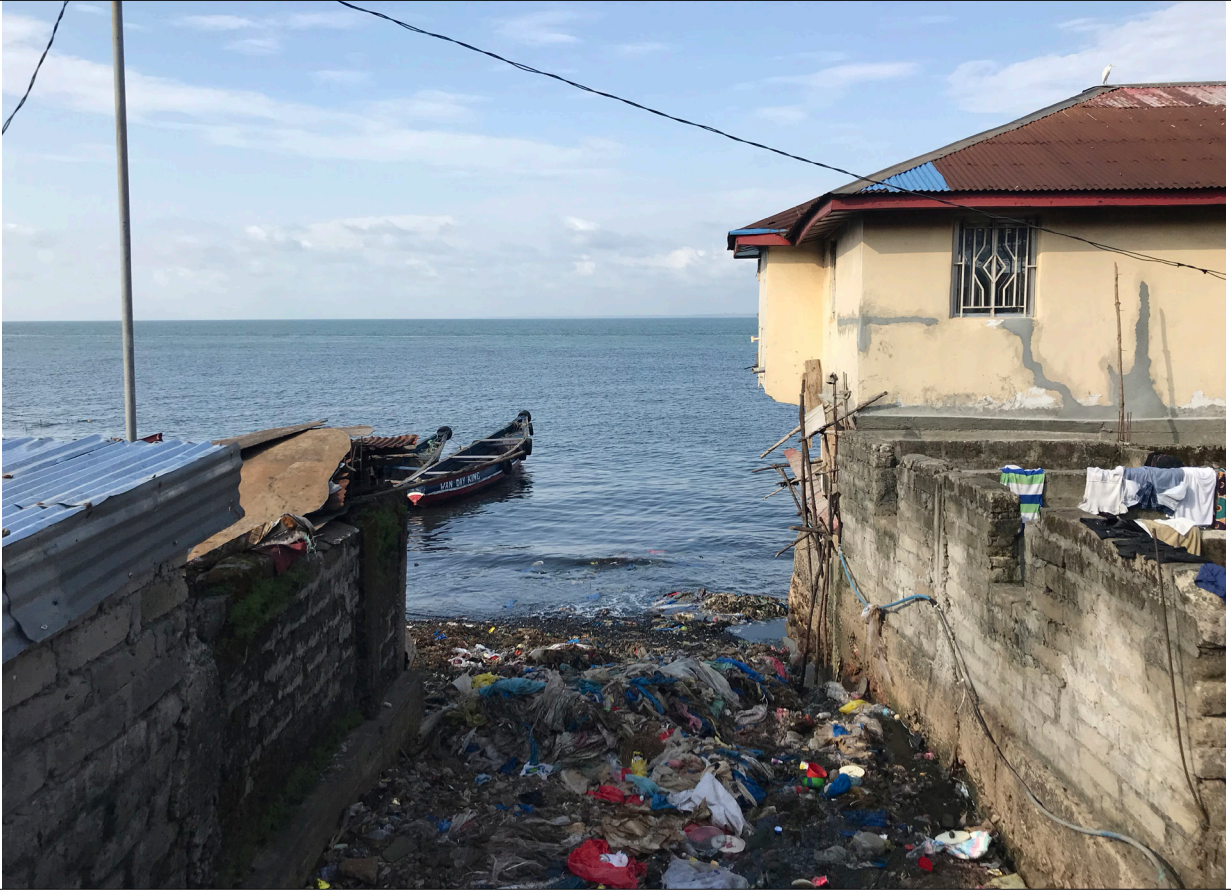
Poor waste management compounds flood risks from harsh storms and sea level rise in Freetown's informal coastal settlements. © Molly Kellogg
