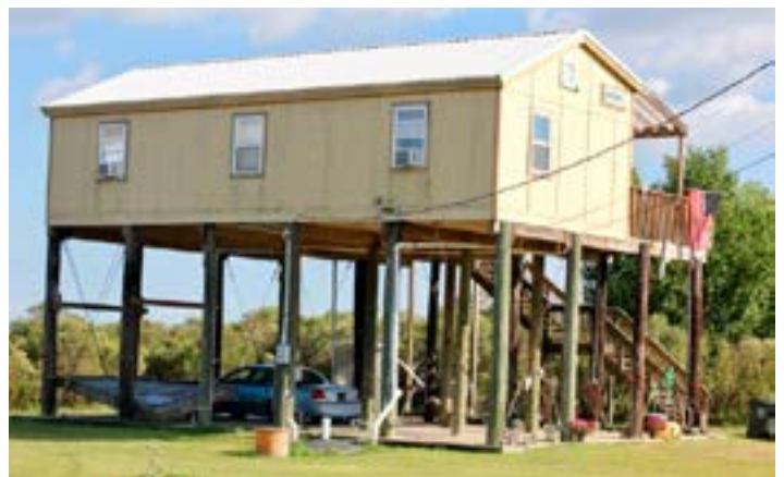
TOP: CHANTEL COMARDELLE IN A LOCAL RESTAURANT. BOTTOM: HOUSE ON STILTS IN ISLE DE JEAN CHARLES, REBUILT AFTER THE LAST STORM. PHOTOS: ERICA BOWER.
